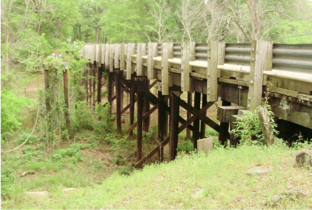
*Figure 7. Bridge 800030 in Grant Parish, built in 1931. Example with five or more spans – 12 main spans (maximum individual span length of 19 feet) comprising an overall length of 223 feet.*
