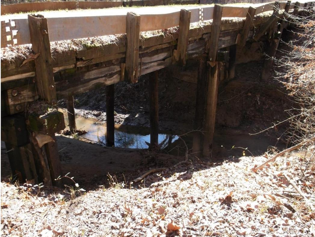
Figure 15. Bridge 600518 in Sabine Parish, 1940. Example of an individual span over 19 feet – four spans comprising an overall length of 77 feet. Longest individual span is 20 feet. See Figure 16 for another view.
