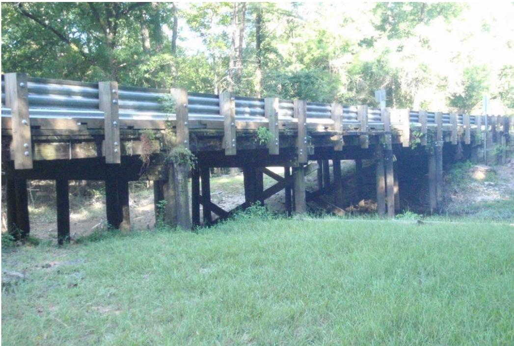
*Figure 12. Bridge 047050 in Caldwell Parish, 1931. Example with five or more spans – five spans comprising an overall length of 97 feet.*
