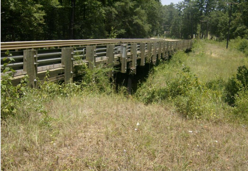
*Figure 9. Bridge 044550 in Vernon Parish, 1944. Example with five or more spans – 10 spans comprising an overall length of 191 feet. See Figure 8 for another view.*
