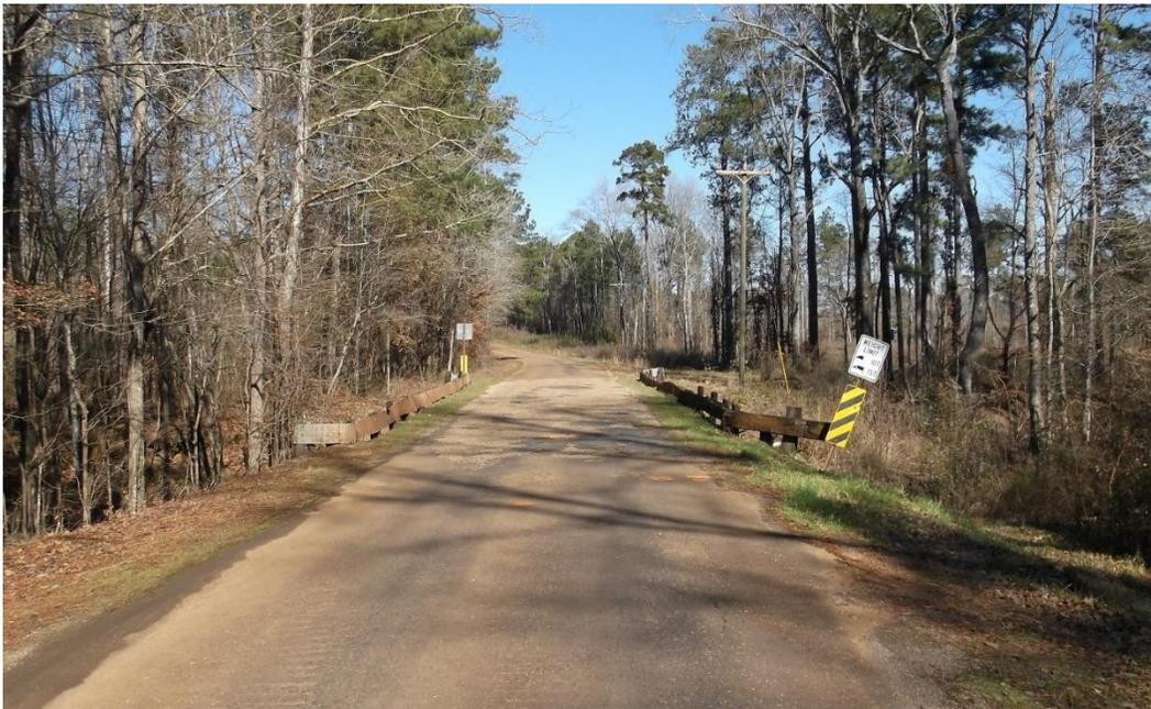
Figure 16. Bridge 600518 in Sabine Parish, 1940. Example of an individual span over 19 feet – four spans comprising an overall length of 77 feet. Longest individual span is 20 feet. See Figure 15 for another view.
