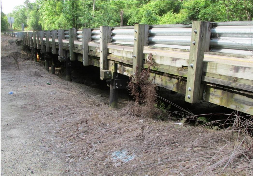
Figure 13. Bridge 065000 in Washington Parish, 1942. Example with five or more spans – five spans comprising an overall length of 97 feet.
