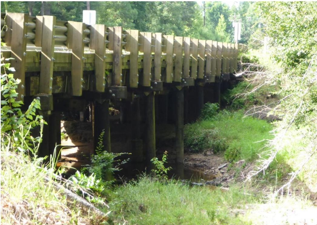
*Figure 8. Bridge 044540 in Vernon Parish, 1944. Example with five or more spans – seven spans comprising an overall length of 135 feet. See Figure 9 for another view.*
