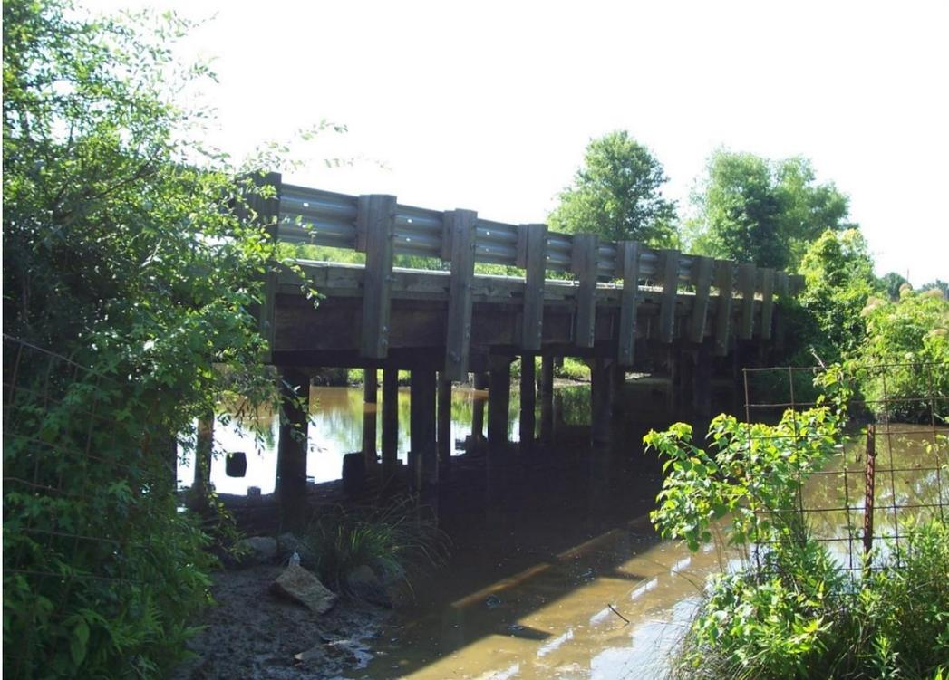
*Figure 6. Bridge 027910 in Union Parish, built in 1936. Example of five or more spans – six main spans (maximum individual span length of 19 feet) comprising an overall length of 115 feet.*
