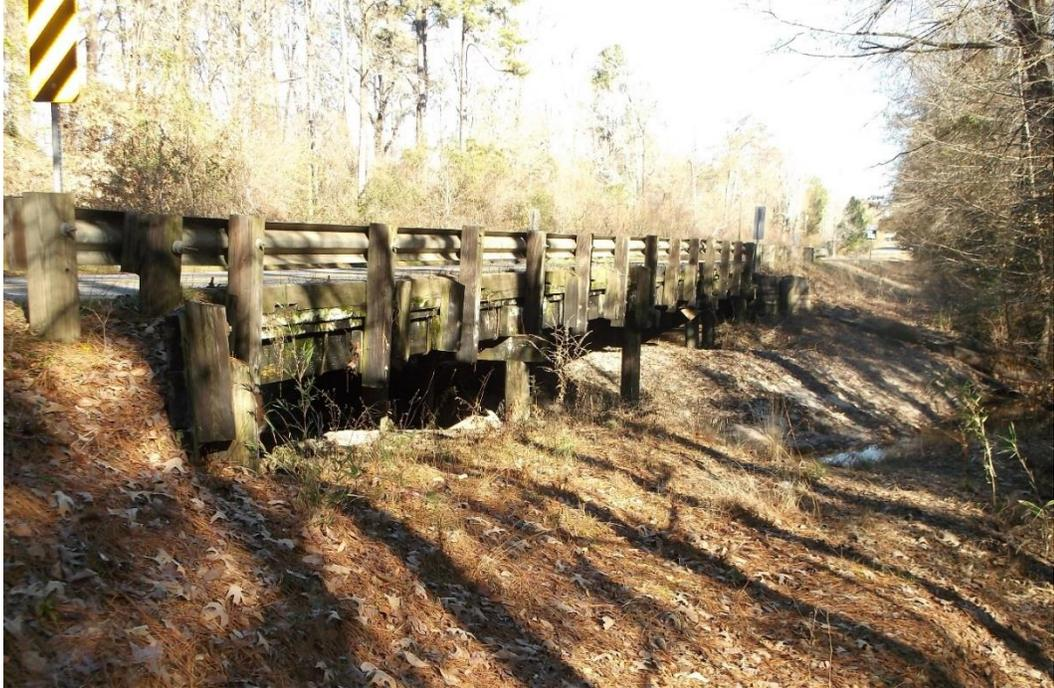
Figure 1. Bridge 038290 in Natchitoches Parish, built in 1926. The bridge has four main spans and an overall length of 78 feet. See Figure 2 for another view.
