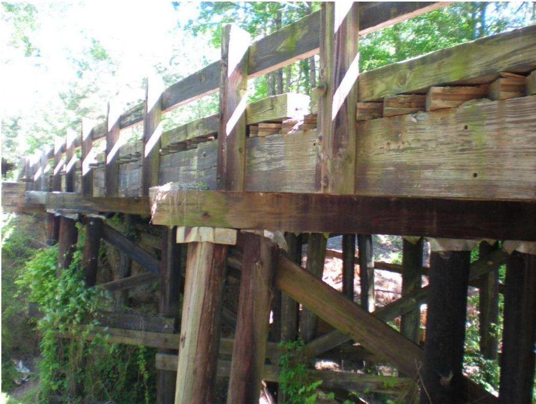
Figure 14. Bridge 400413 in Ouachita Parish, 1942. Example with five or more spans – five spans comprising an overall length of 80 feet.
