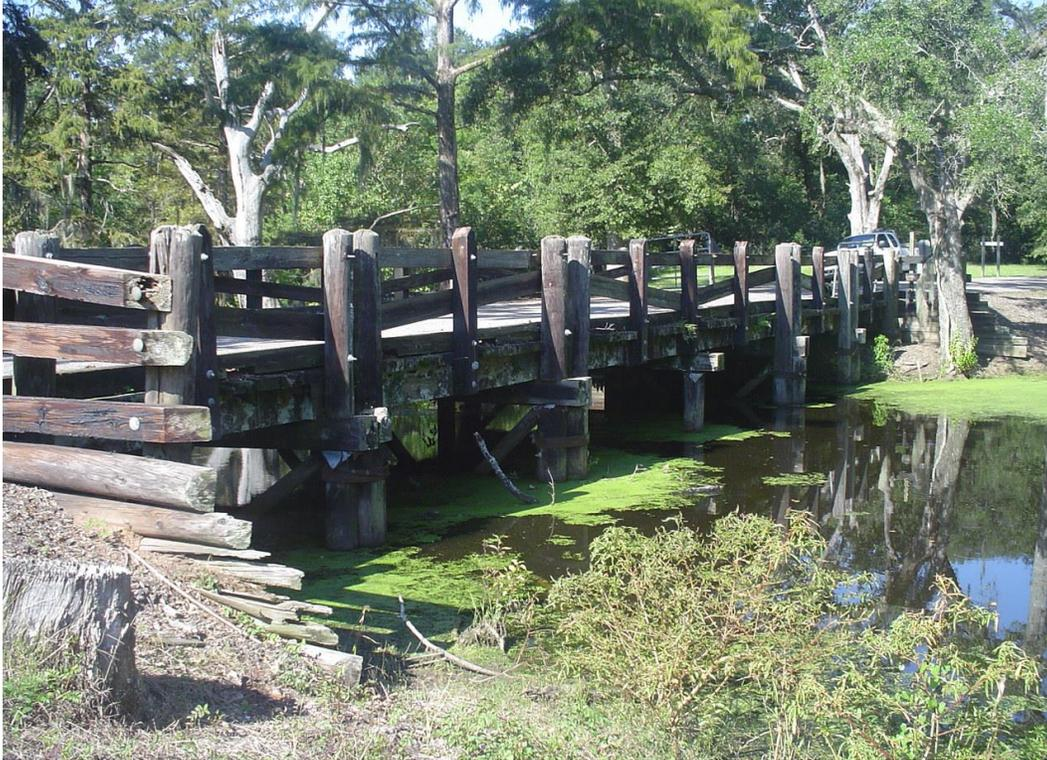
*Figure 3. Bridge 008900 in St. Martin Parish, 1938. This bridge has five main spans, with the longest individual span—29 feet—within the study pool. Overall length is 86 feet.*
